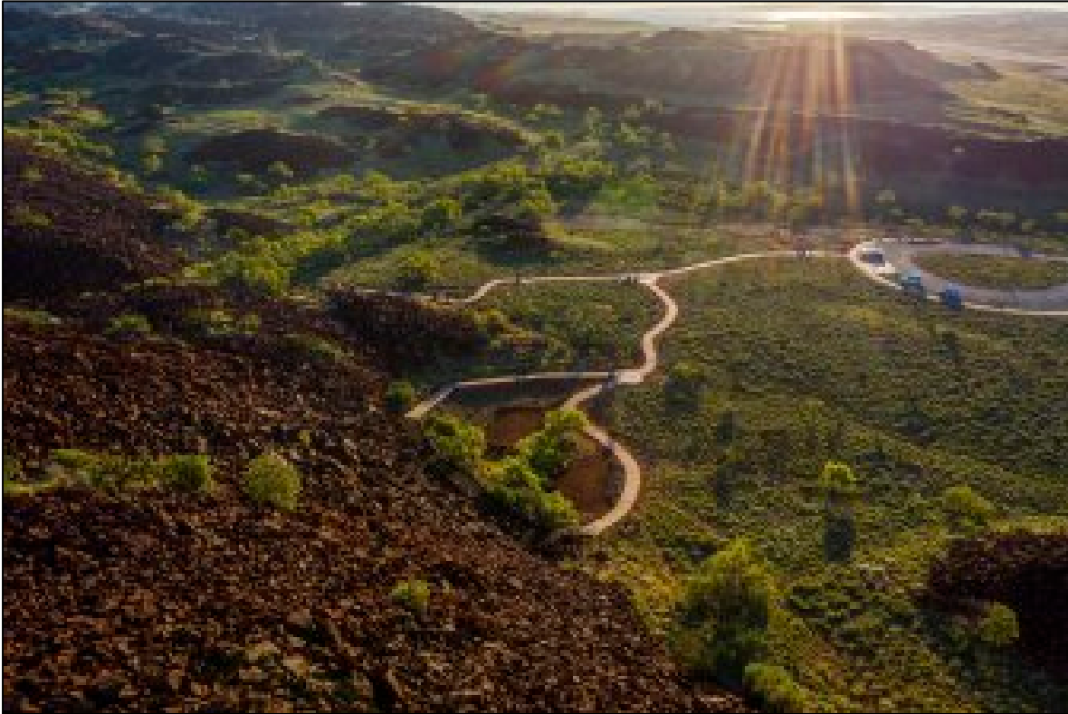
New boardwalks for the Murujuga rock art cultural tour.
