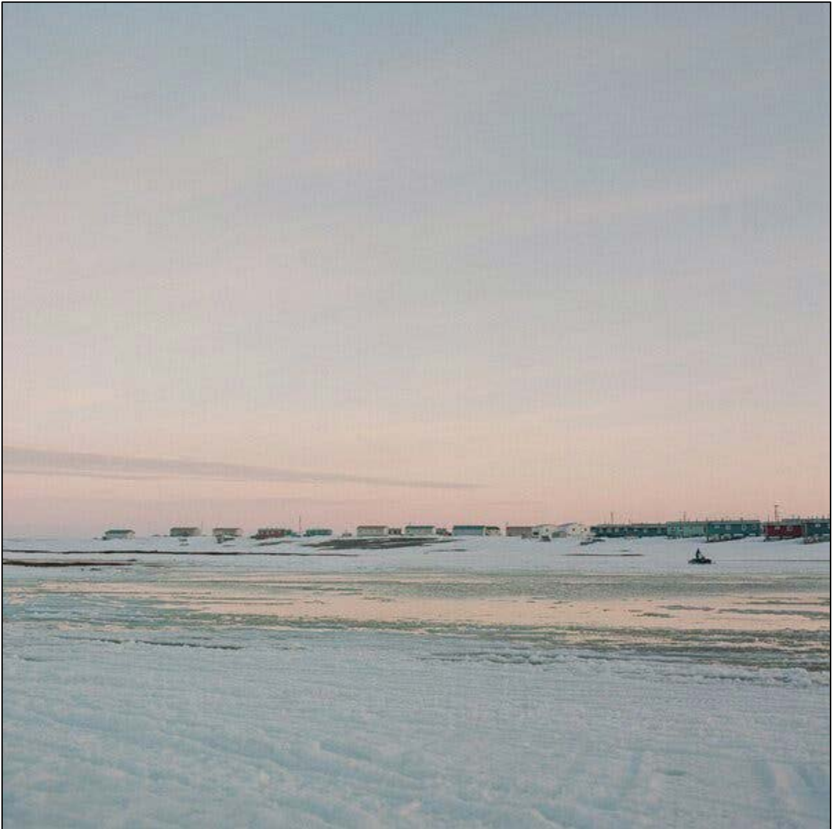
Chefnak, Alaska, where the foundations of many buildings are failing as the permafrost thaws, in April. Credit...Ash Adams for The New York Times
